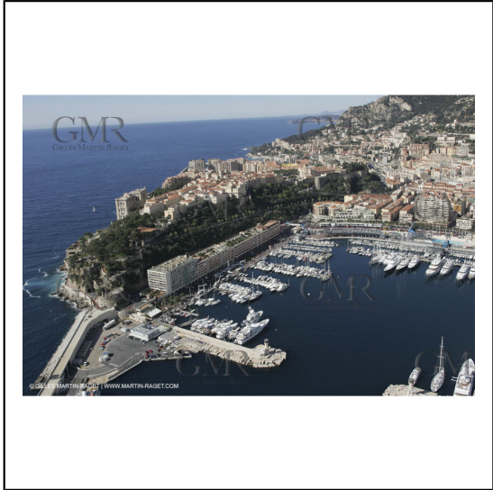
Monaco - Installations Monaco Marine***Monaco - Monaco Marine settings
