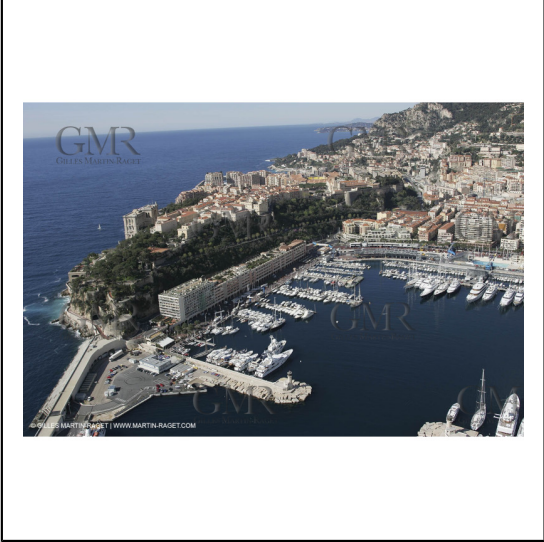
Monaco - Installations Monaco Marine***Monaco - Monaco Marine settings
