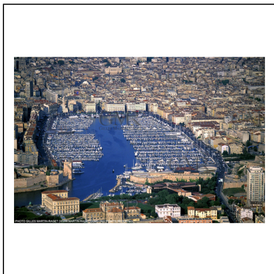
Vieux Port***Old harbour
