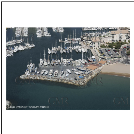
Fréjus - Installations Monaco Marine***Fréjus - Monaco Marine settings
