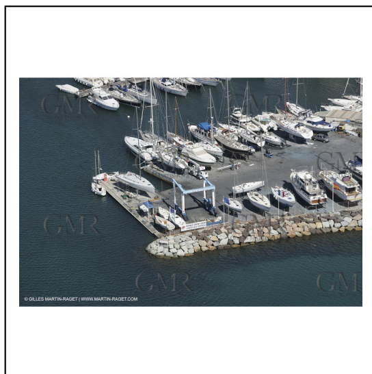
Fréjus - Installations Monaco Marine***Fréjus - Monaco Marine settings
