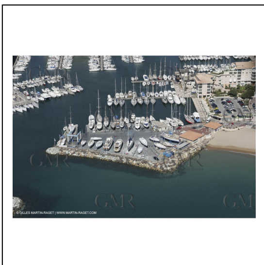
Fréjus - Installations Monaco Marine***Fréjus - Monaco Marine settings
