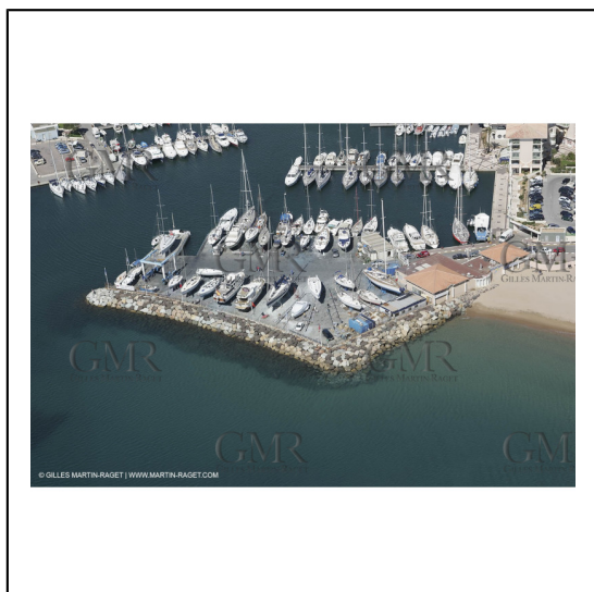
Fréjus - Installations Monaco Marine***Fréjus - Monaco Marine settings
