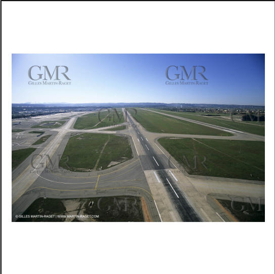
Etang de Berre (FRA,13) - Aeroport de Marseille-Provence***Berre Lake (FRA,13) - Marseille-Provence Airport
