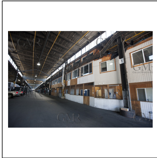
07/06/2011 - San Francisco (USA,CA) - 34th America's Cup - The Piers in their state of origin - Pier 23
