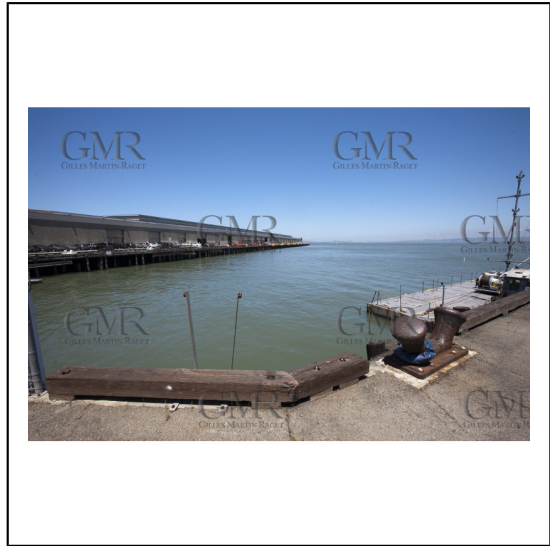
07/06/2011 - San Francisco (USA,CA) - 34th America's Cup - The Piers in their state of origin - Pier 23
