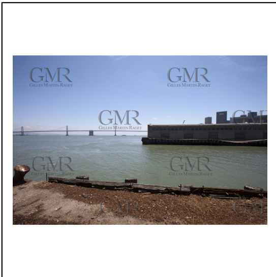
07/06/2011 - San Francisco (USA,CA) - 34th America's Cup - The Piers in their state of origin - Pier 23
