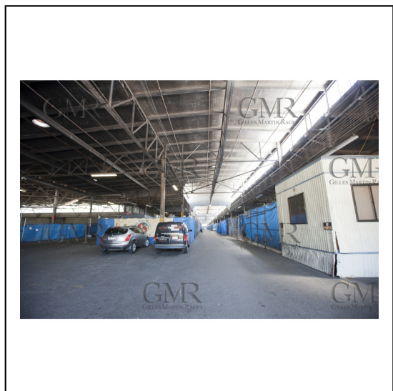
07/06/2011 - San Francisco (USA,CA) - 34th America's Cup - Event sites - The Piers in their state of origin - Pier 19
