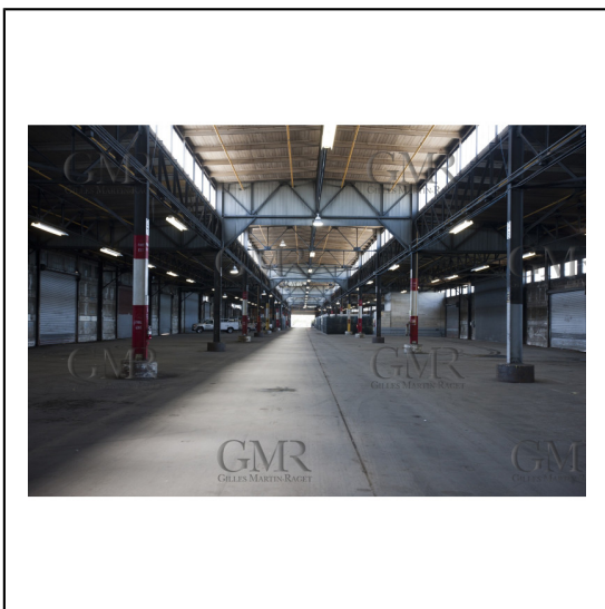
07/06/2011 - San Francisco (USA,CA) - 34th America's Cup - The Piers in their state of origin - Pier 23
