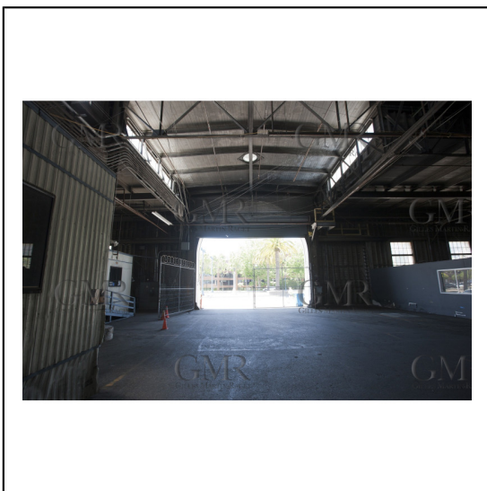
07/06/2011 - San Francisco (USA,CA) - 34th America's Cup - Event sites - The Piers in their state of origin - Pier 19
